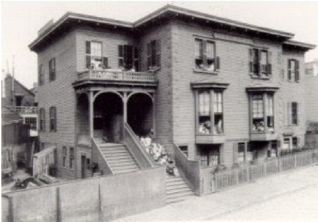
Figure 4. Silver Street Kindergarten, 64 Silver Street, near Third, ca. 1879. Source: CA.gov, "19th Century Kindergarten Uncovered in San Francisco," at https://dot.ca.gov/caltrans-near-me/district-4/d4-popular-links/forward-issue-3/kindergarten , accessed 7-17-23.
